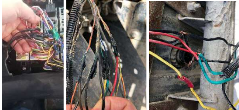
Improper cable connection examples
